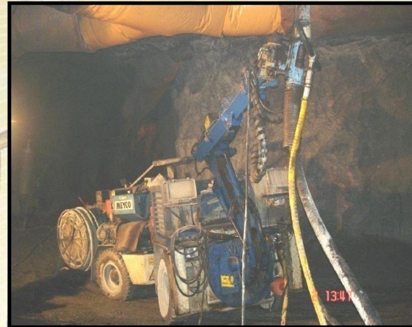
MEYCO robot spraying concrete in the gallery
